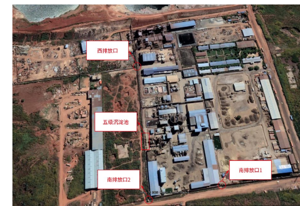
Satellite image of CDM plant sedimentation tank and discharge outlets
