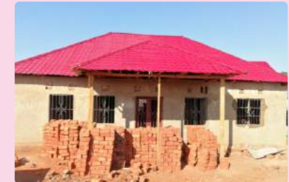
House after renovation
