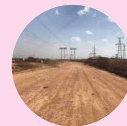
KASAPA road repaired by CDM
