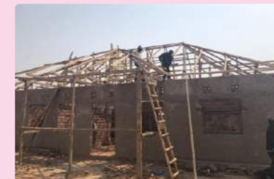
House under construction
