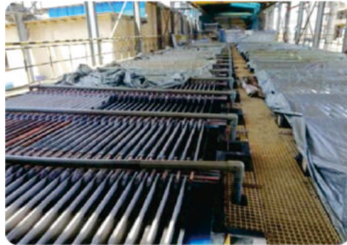
Completed installation of acid gas recovery pipeline
