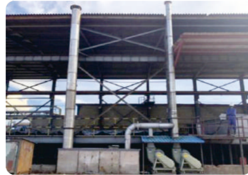
Completed installation of acid mist fan
