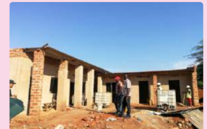
Police station after renovation
