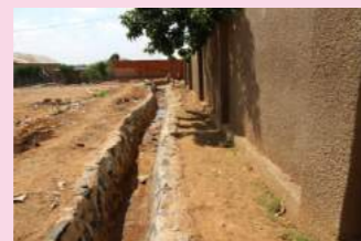
Drainage ditch in the Village
