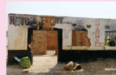
Pharmacy before renovation
