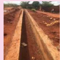
Drainage ditch in KAMATETE
