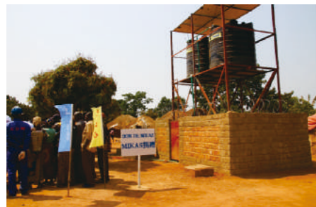
MIKAS-funded Solar Water Well in Village
